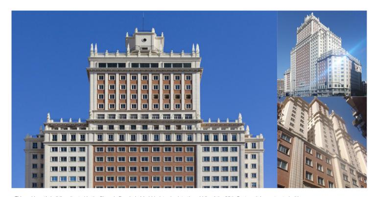
This emblematic building situated in the Plaza de España in Madrid, dates back to the middle of the 20th Century. It is constructed with reinforced concrete perimeter walls and columns which employed smooth rebar. The horizontal structure is composed of one-way slabs resting on reinforced beams with the same rebar type. The foundation unit is composed of surface rectangular-shaped footings which taper and stagger upwards.
